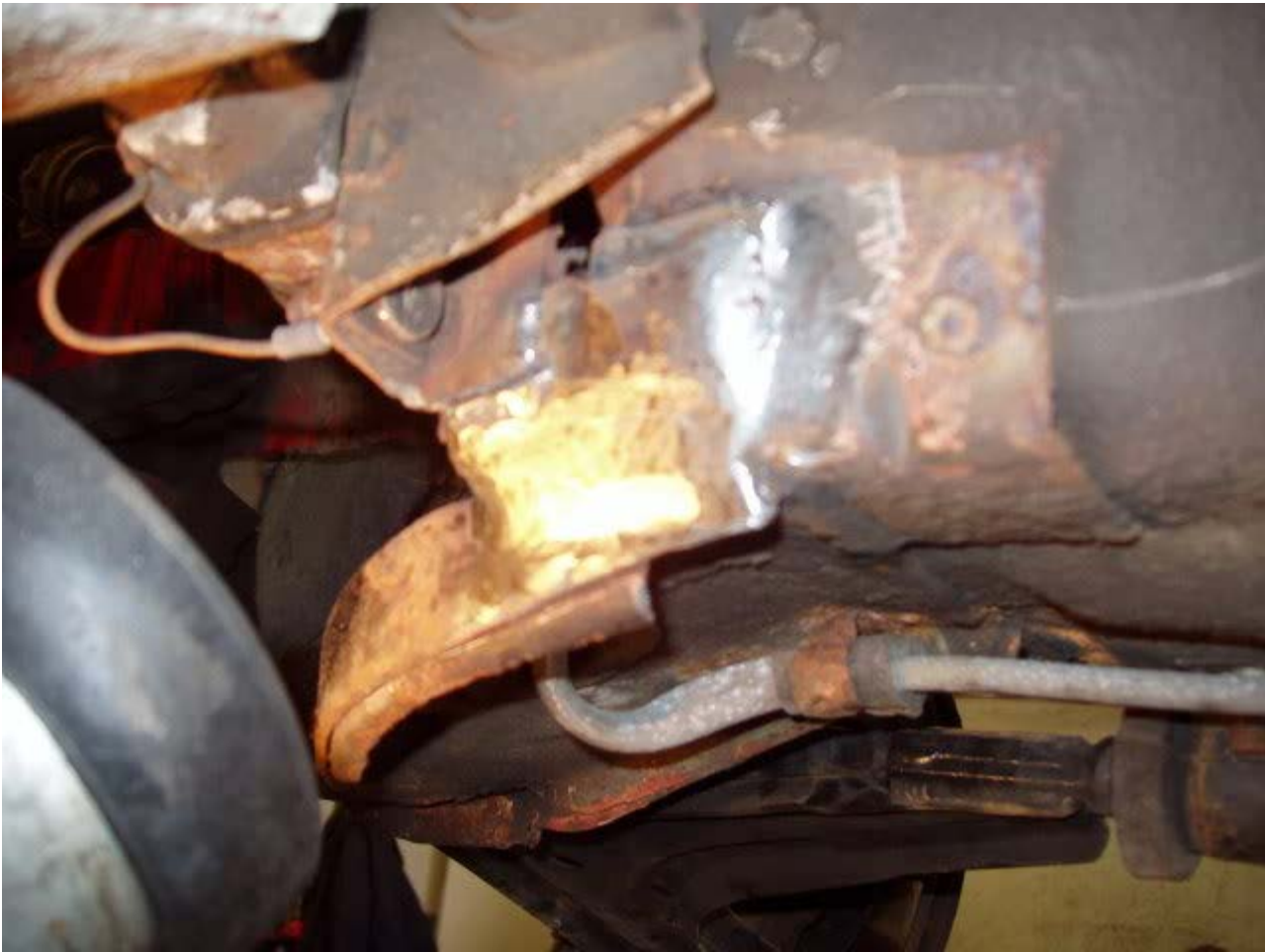
proper job!!! all welded back together, then undersealed
